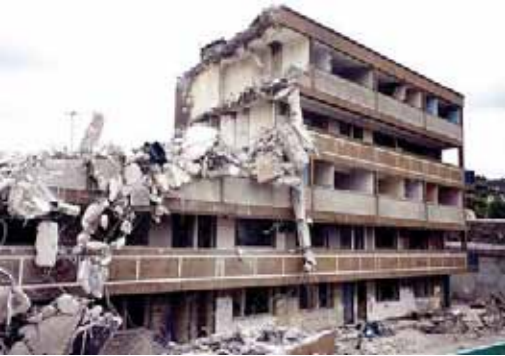
The former Glen Flats during demolition.
