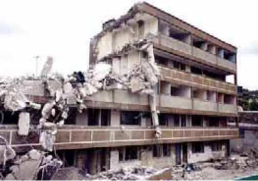
The former Glen Flats during demolition.
