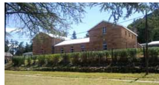
The Community Centre in Hardenburg which contains a respite centre, consulting rooms, a dispensary, ablution offices, catering facilities and waiting areas for residents.
