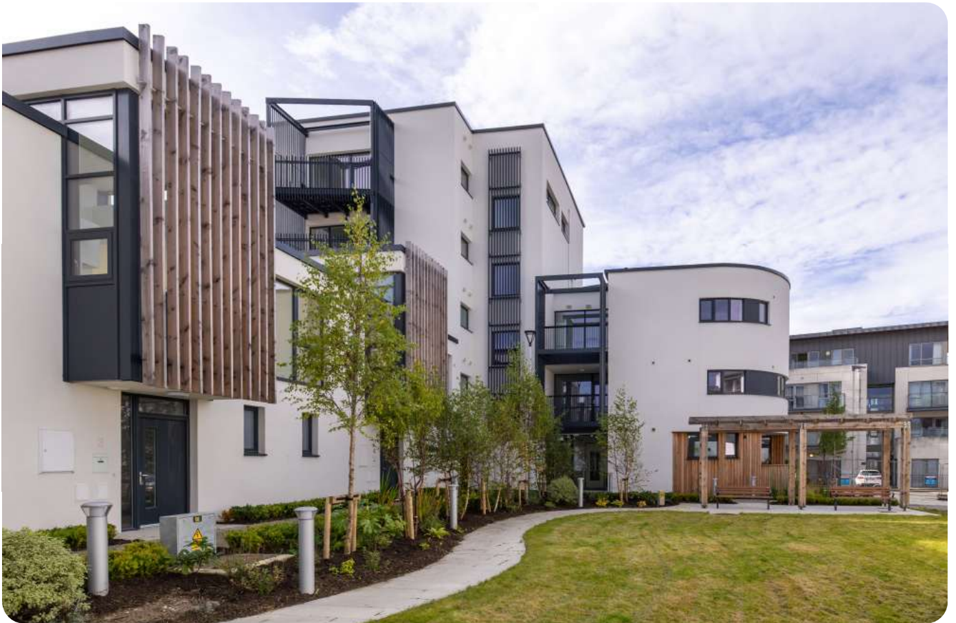
Fig.236. Building quality homes Beechpark, Respond, Donnelly Turpin Architects
