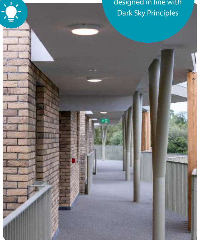
Fig.102. Walkway lighting Carrs Lane, Respond, Opperman and Associates
