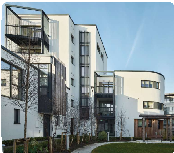
Fig.101. Clear wayfinding through strong landscape design Beechpark, Respond, Donnelly Turpin Architects
