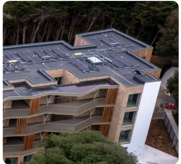
Fig.152. Rooftop plant Carrs Lane, Respond, Opperman and Associates
