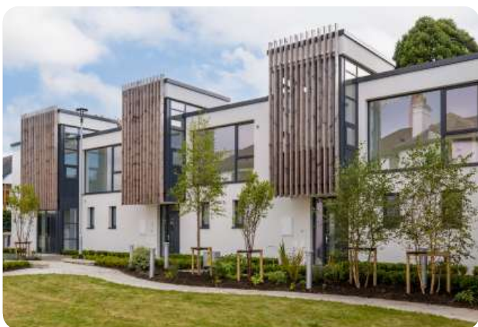
Fig.225. Careful placement of soft landscaping Beechwood, Respond, Donnelly Turpin Architects
