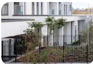
Fig.165. Safe and secure roof terraces Charlestown, Respond, MCORM Architects
