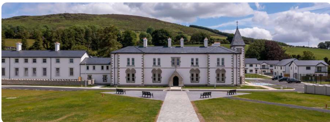
Fig.103. Street lighting, communal gardens and visual connections Baltinglass, Respond, PD Lane Associates
