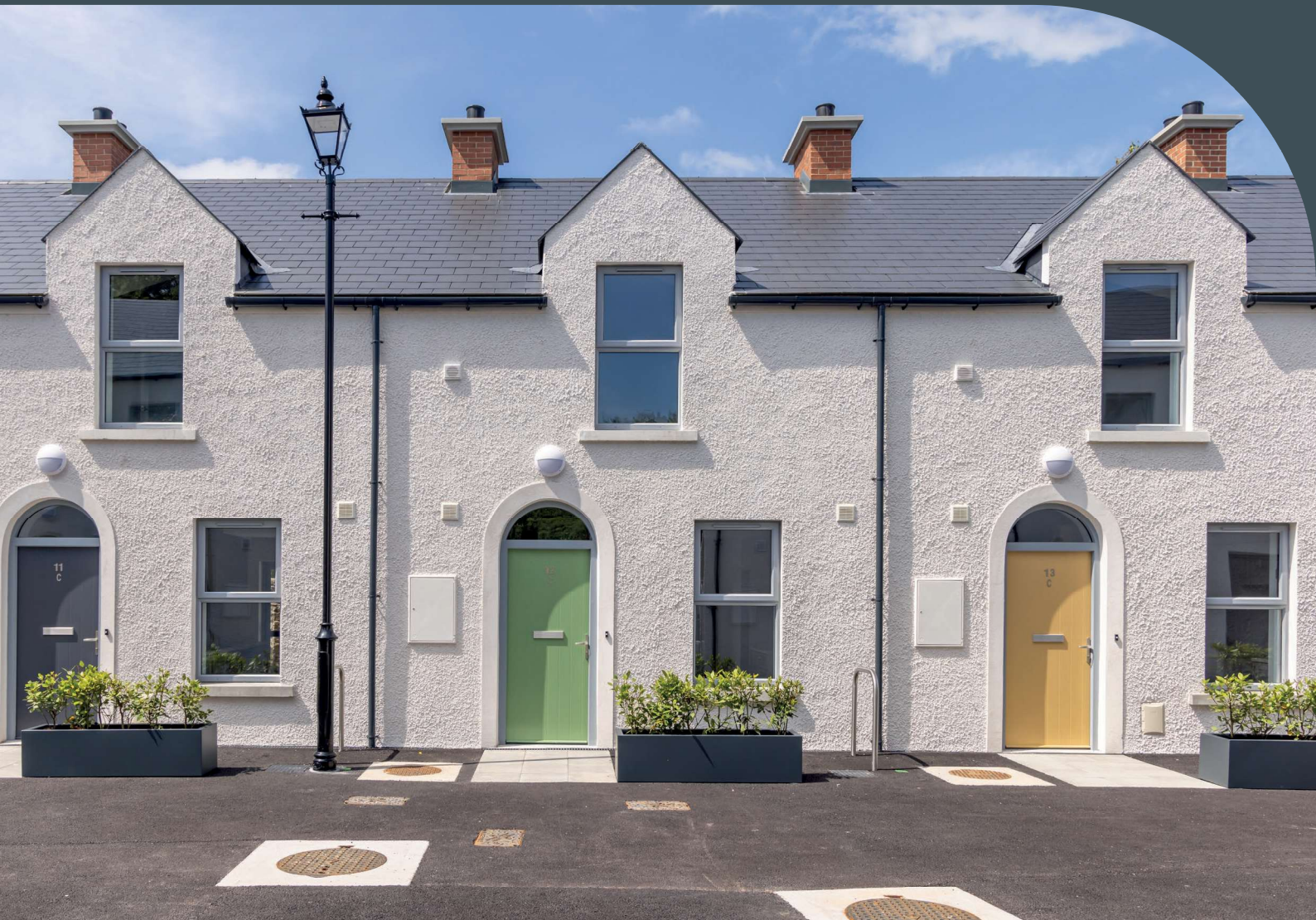
Fig.2. Millfield Cottages Cork, Respond, CBA Architecture
