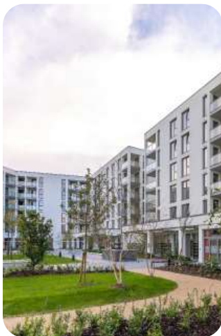
Fig.164. Overlooked shared space Charlestown, Respond, MCORM Architects
