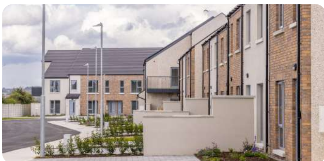
Fig.83. Threshold between homes and access walkways Brindle Close, Kilbarry, Respond
