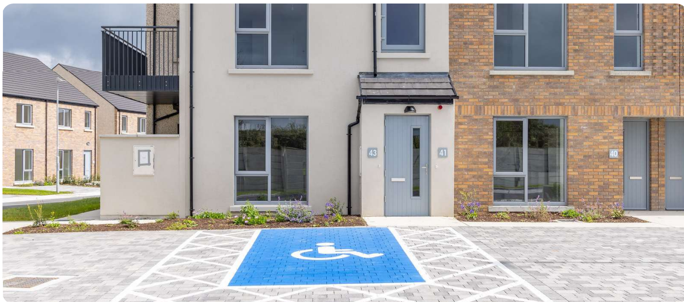
Fig.82. Residential Threshold considering access for all and car parking Brindle Close, Kilbarry, Respond
