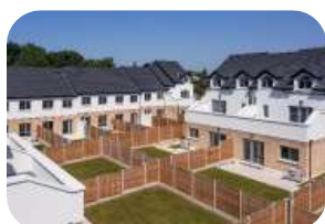
Fig.87. 1.8m timber fences Old Corduff, Respond, Crawford Architecture
