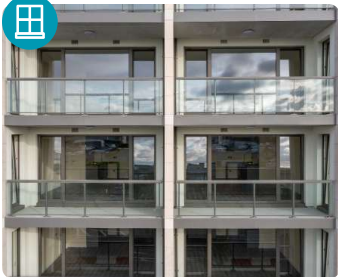
Fig.109. Windows accessed by balcony for cleaning Charlestown, Respond, MCORM Architects
