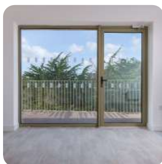
Fig.174. Balanced window proportions Carrs Lane, Respond, Opperman and Associates
