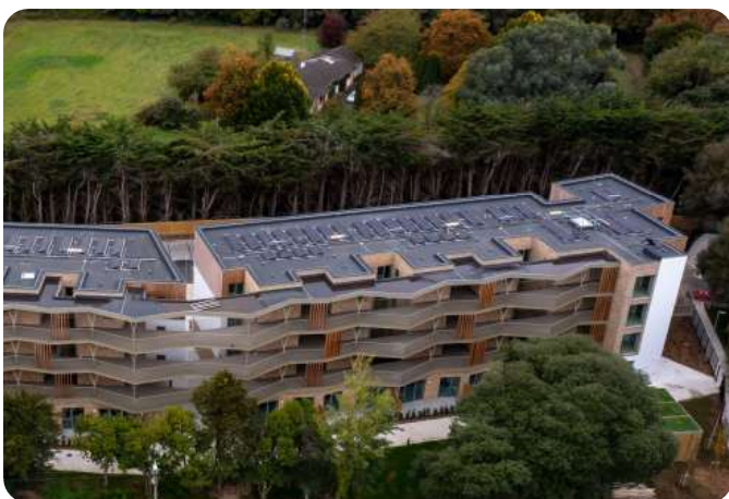
Fig.229. Roof access and safety systems Carrs Lane, Respond, Opperman and Associates
