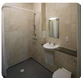
Fig.181. Level access shower Hazelhurst Court, Levitt Bernstein
