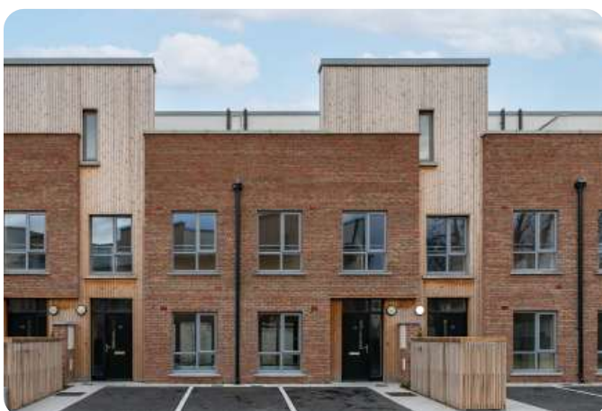
Fig.110. Low level windows can be cleaned by pole Kingswood, Respond, Crawford Architecture
