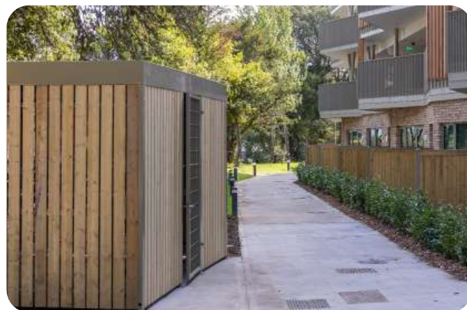
Fig.108. Communal bin store Carrs Lane, Respond
